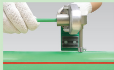
Repairing stick welding
